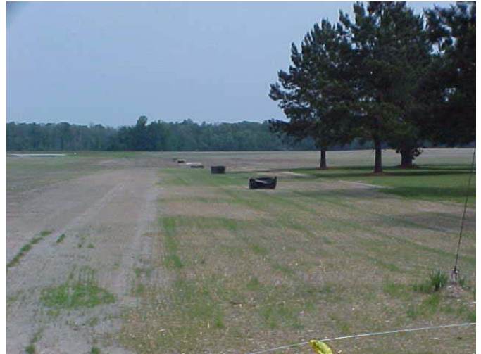
Photo: Installation of Storm Drainage Facilities
