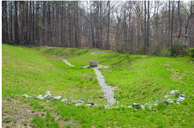
Example of a dry detention basin.
